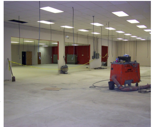
Progress Drive is being remodeled
